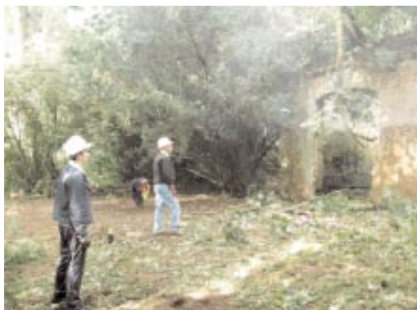
In June 2003, a tree fell on the O'Neill's summer house and caused considerable damage. After discussion with Lord O'Neill and the Natural and Built Heritage of the Environment and Heritage Service, it was decided to remove the tree from the house, and the trees growing out of and around the house. This was all done by volunteer members, among them was vice-president Brian Cassells, seen here on the right
